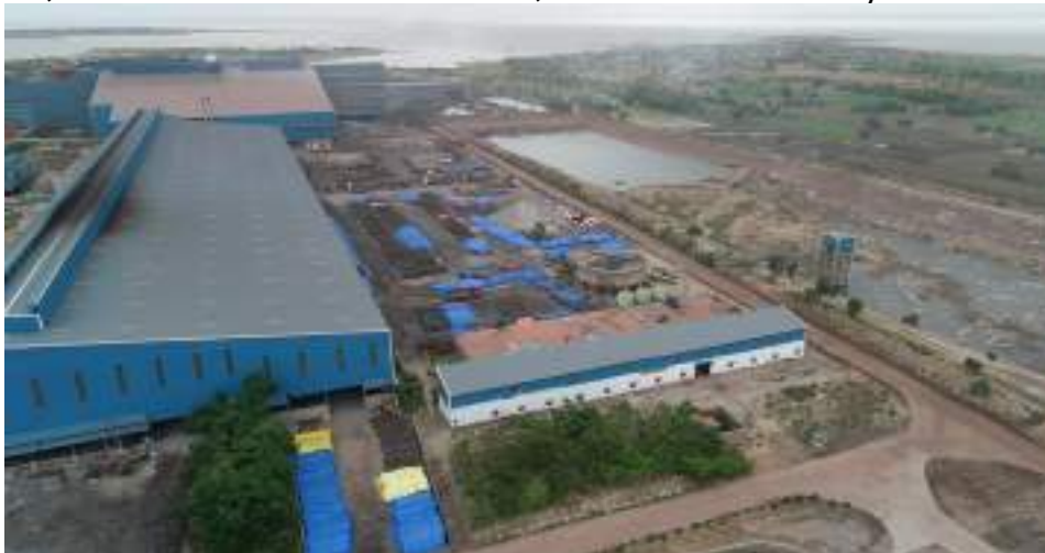
RMS, RAW WATER TREATMENT UNIT, PPC STOCK YARD & N/E RESERVOIR
