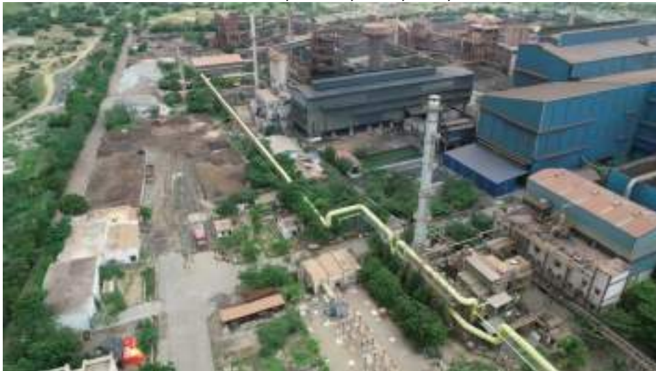
PIG IRON STOCK YARD, RMHS, MBF, CPP, FIRE STATION
