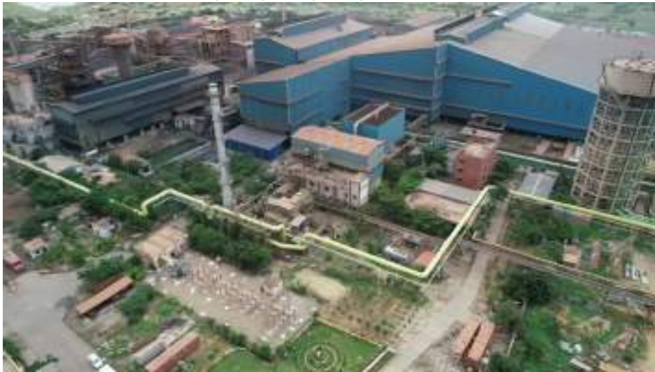
OLD MRSS, CPP, MBF, SMS, OVER HEAD TANK.
