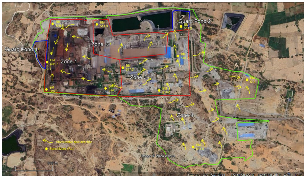
Fig. 3: Google earth map showing radial mirco drainage pattern guard ponds and storm water flow zones
