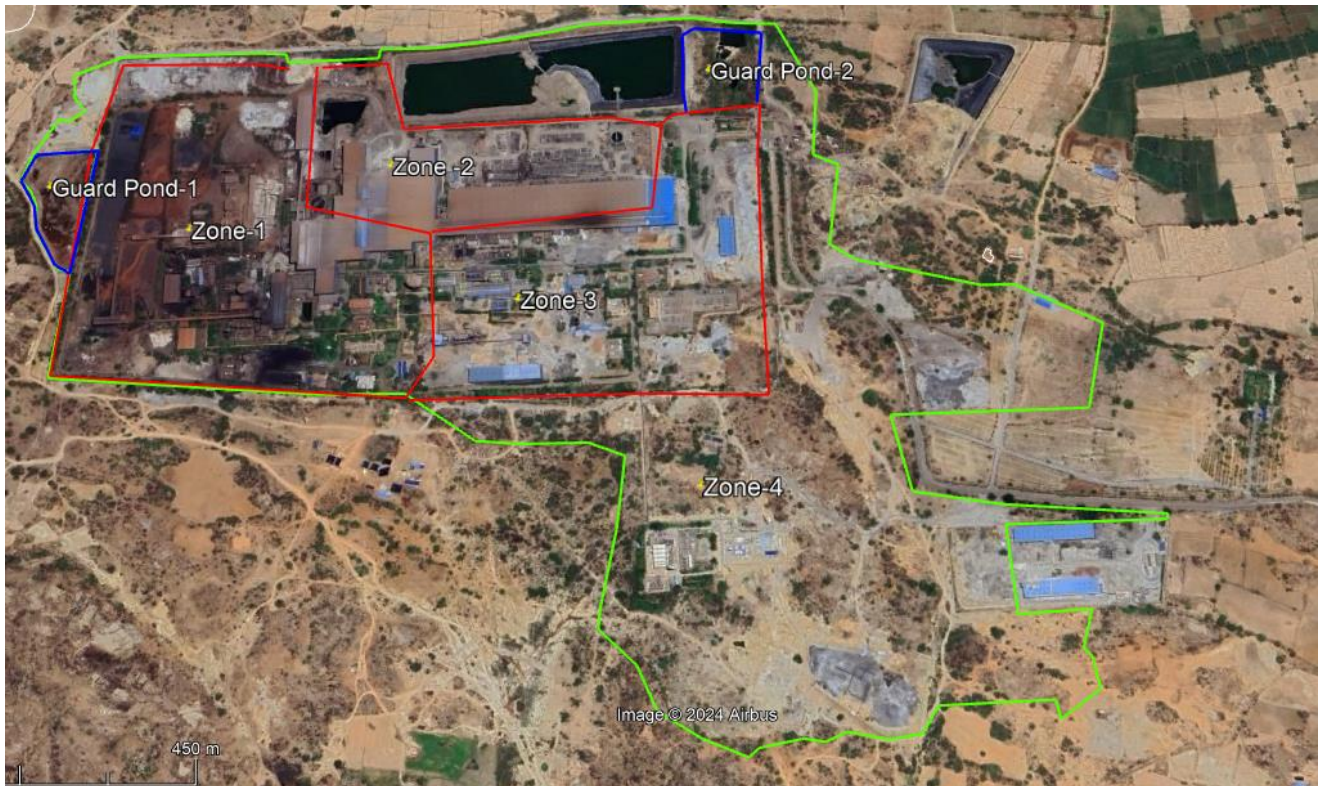
Fig.3: Google earth Map showing different zones of topography draining storm water and guard ponds 1 & 2.
